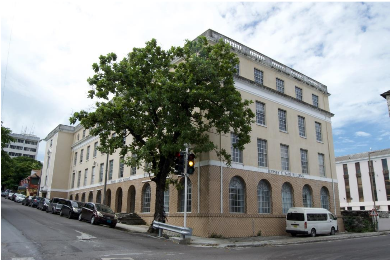
View of Rodney E. Bain building from Shirley Street (2020).
