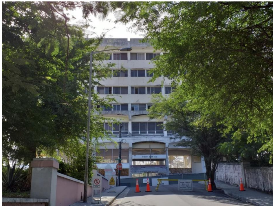
Post Office building during demolition (2021). View from Parliament Street.
