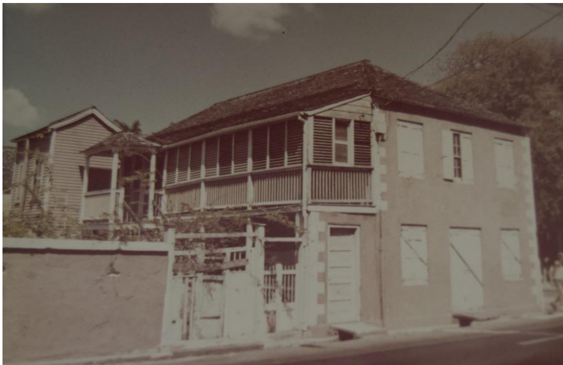
Magna Carta Court building prior to removal of plaster, circa 1979. Photo courtesy of Lori Lowe.
