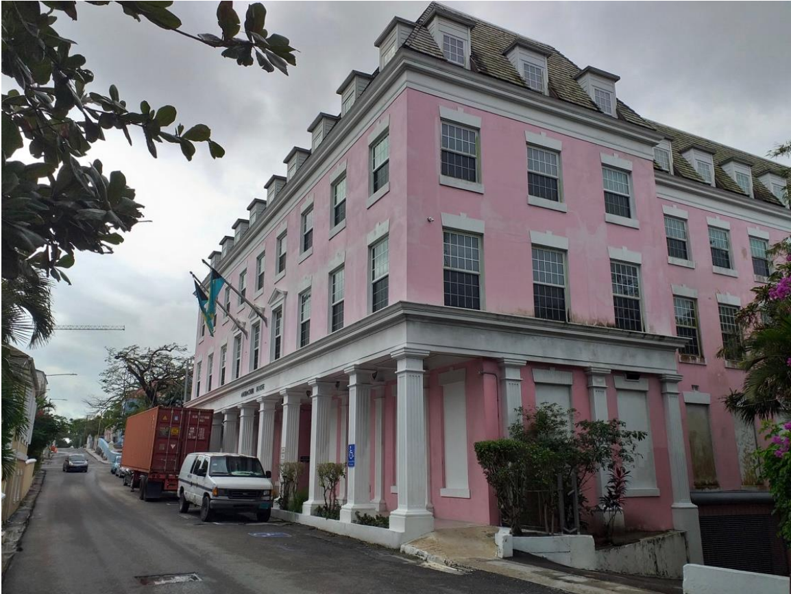
Ansbacher House building (2021). View from East Street.
