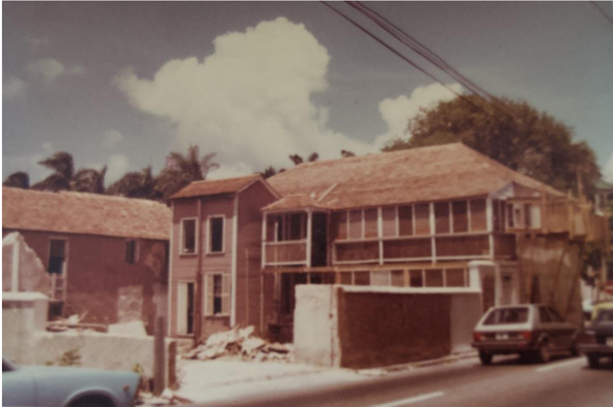
Magna Carta building during renovations, circa 1980. Photo courtesy of Lori Lowe.
