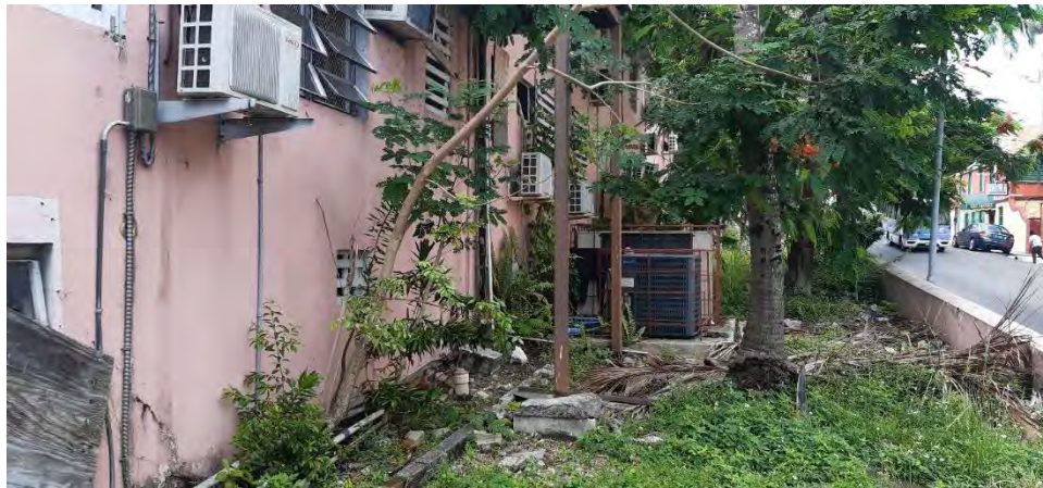
Figure 47. West side of HIV Centre, facing south along Parliament Street .
