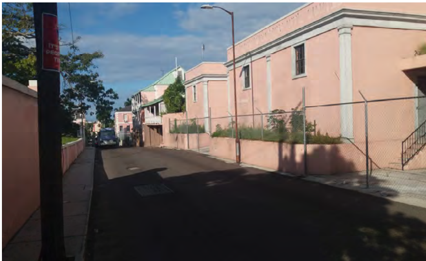
Figure 4 (East Street Looking North)
