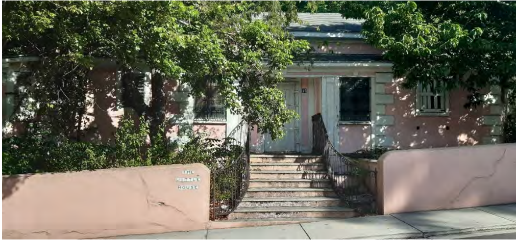
Figure 92. Images of LS1 located at the western entrance of The Little House
